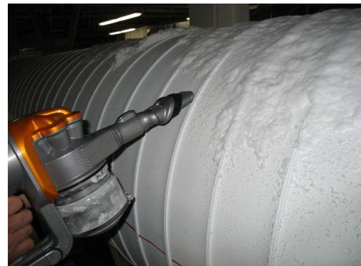
Figure 4 – Using portable vacuum to collect dust from round duct work
