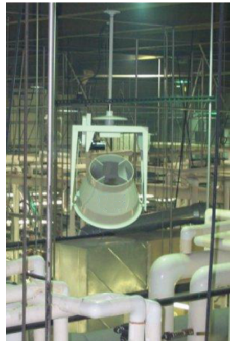
Figure 6 – Oscillating Fan Installation
